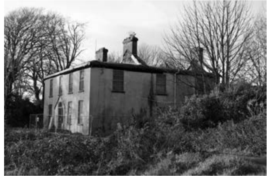
Fig. 9: Beechgrove House following the fire, view from the southeast (Photo: author).
