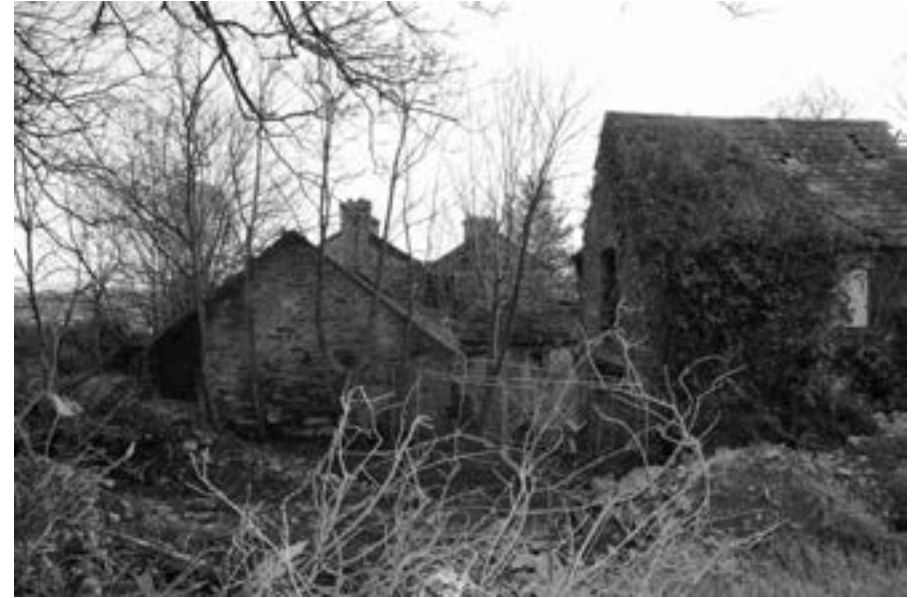
Fig. 11: Various outbuildings to north and east of Beechgrove House (Photo: author).
