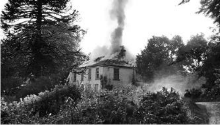
Fig. 1: Fire in Beechgrove House, 16 June 2017 (Photo: courtesy of Dr Jason Van Der Velde of West Cork Rapid Response).
